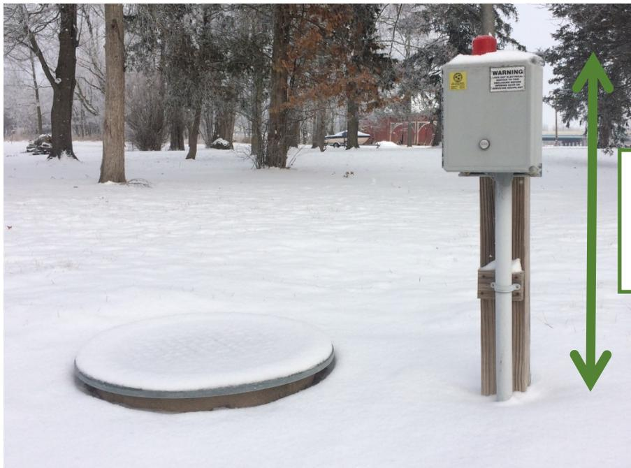
The Control Panel for an individual grinder pump station is approximately 24" to 36" tall.
